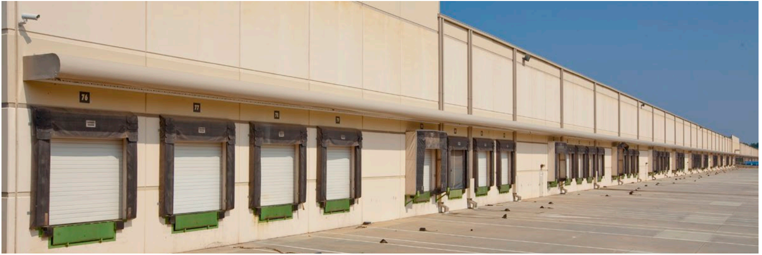
Dock injuries cost distribution centers money and good employees. As a result, more effort is going into designing safer work environments for dock employees. Included in these changes are installing pneumatic or hydraulic levelers, vehicle restraints, and LED lights.
