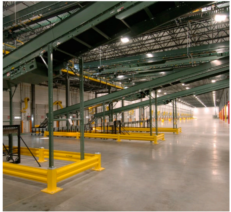
As companies struggle to reduce costs, more warehouses are incorporating energy efficient design elements to cut operating costs.
